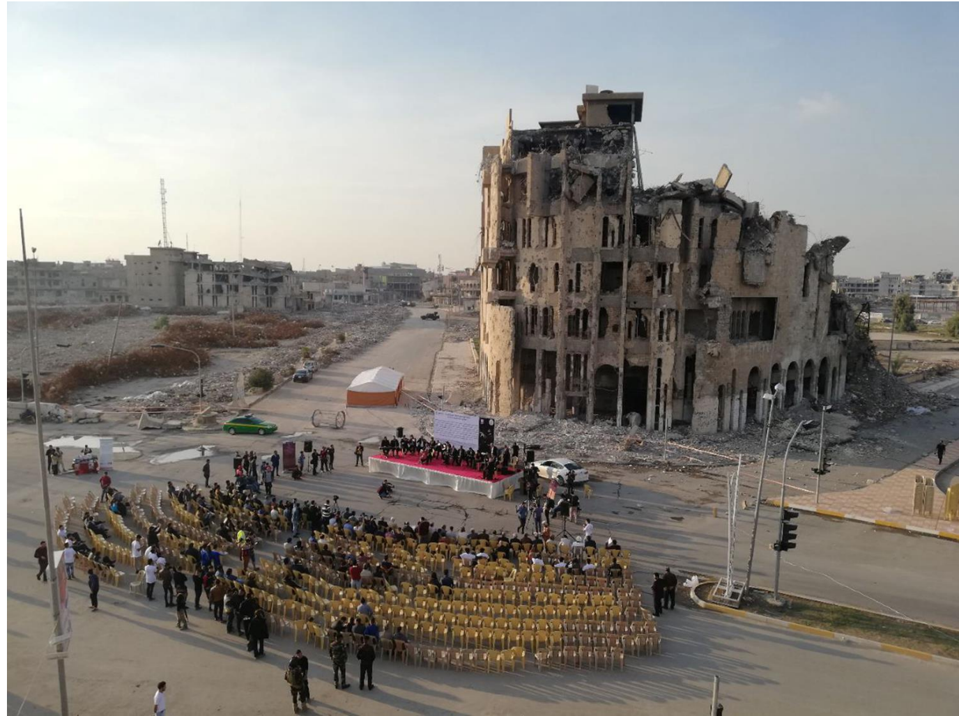
Insurance Building, Al Gumhorya Street, Al Taameen, Old City, Mosul, Iraq 2018
