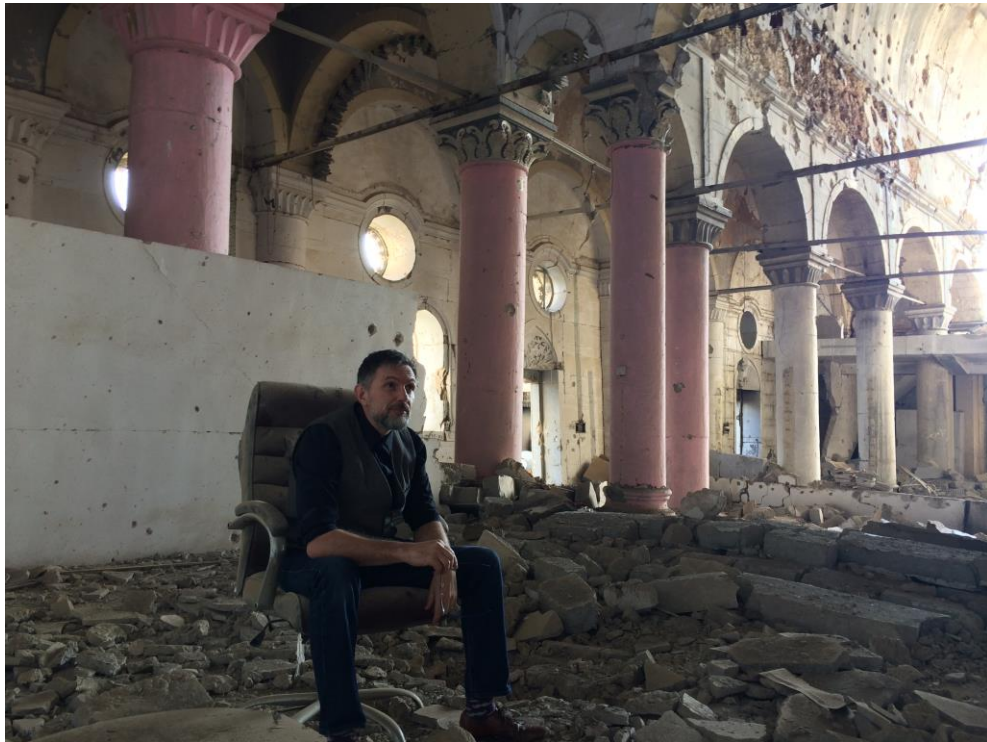
Tahira Church, Mosul. Iraq 2017 I entered al-Tahira church, through a small door covered in graffiti we found heaps of ISIS-designated contraband, bodies, graffiti and plenty of rubble alongside signs that the building had been used for something more sinister. I learnt from a local teacher, his brother and many others that this church had been a prison and punishment facility, it had been run by the dreaded Hisbah in Mosul. It was a place feared by the local community, a place many didn't come back from
